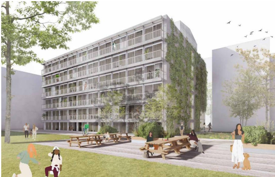
Figure 4. North and west facade of Maria Austriastraat
