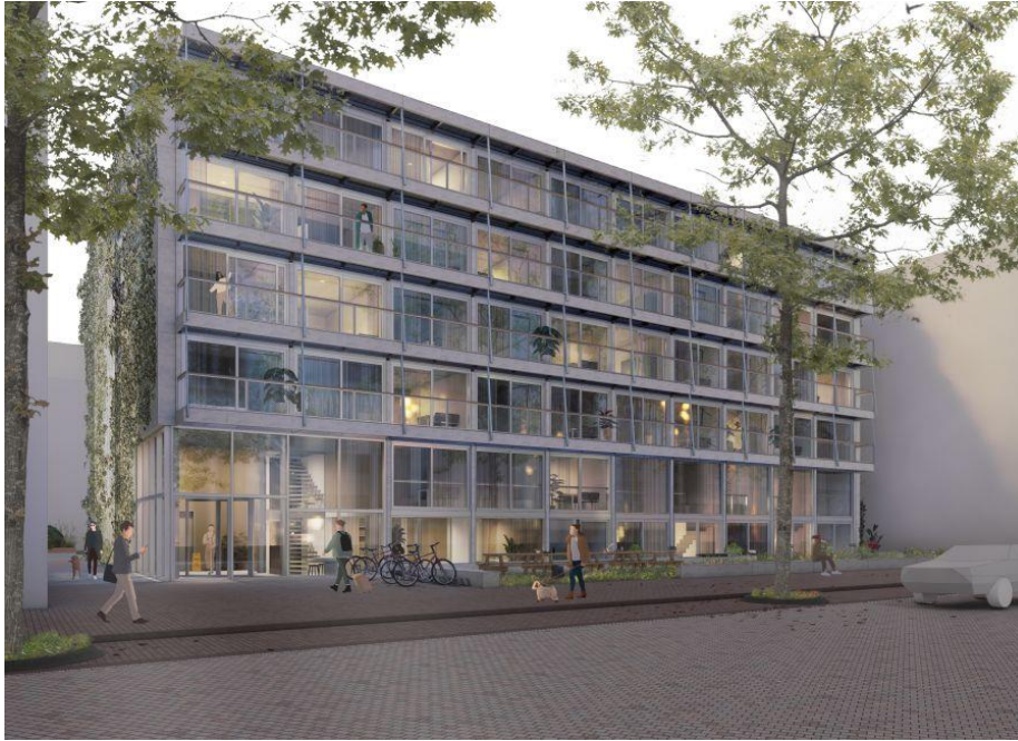
Figure 3. South facade of the Maria Austriastraat
