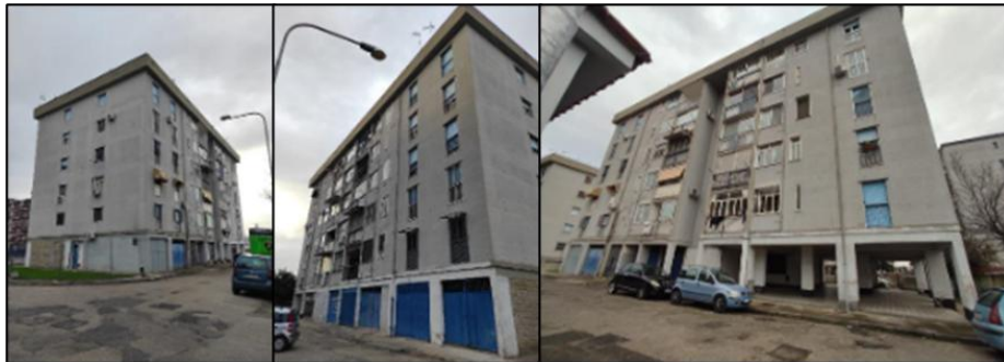
Figure 1. The Acerra demonstrator from outside.
