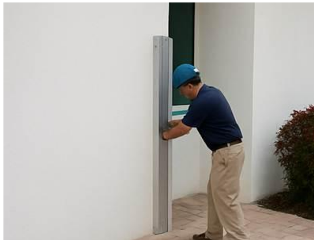
Figure A 3. Installing side bars attached to the building
