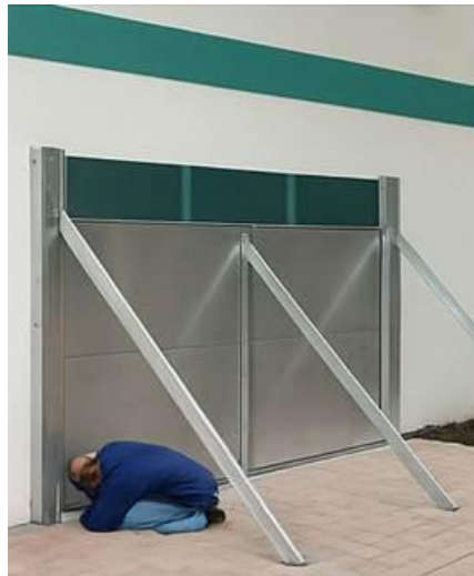
Figure A 5. Fixing braces for stability
