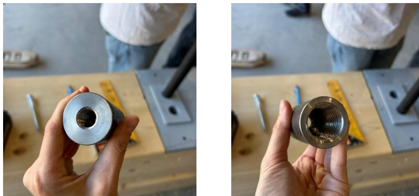
Figure 21. Example of steel couplers for bolts and dissipaters
