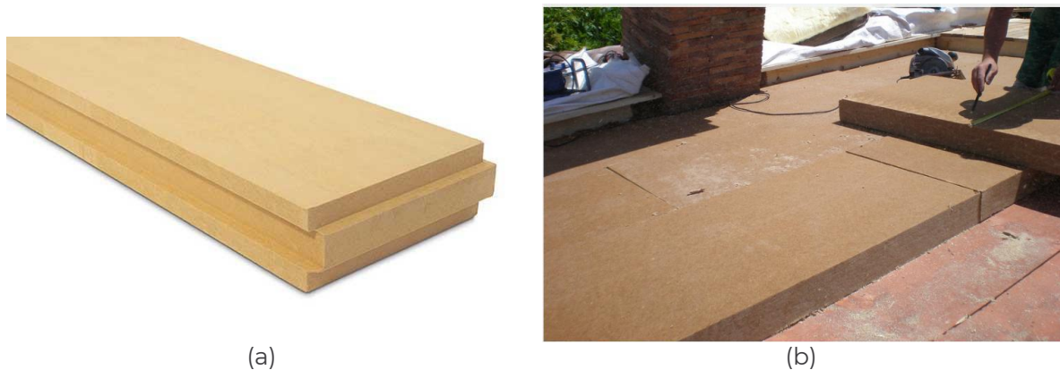
Figure 13. Roof insulation: (a) timber-fibre insulation panels and (b) example of in-situ installation (images available online: https://www.betonwood.com/ ).
